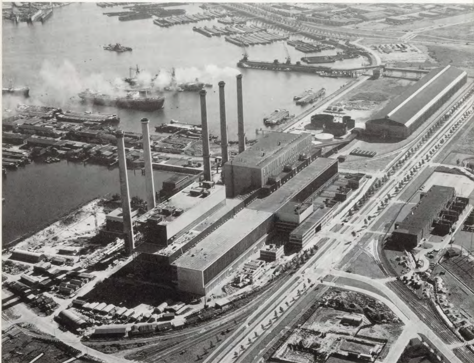
Figure 1 - Electric power plant 'Waalhaven' at Rotterdam. Enlargement under construction. (Photo KLM Aerocarto N.V.).
