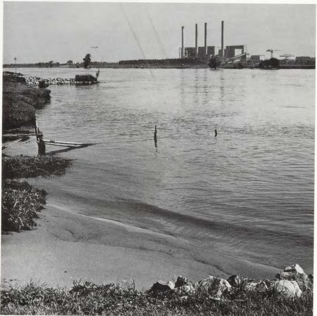
Figure 5 - Electric power plant 'IJsselcentrale', at Harculo (Photo Jan van de Kam)
