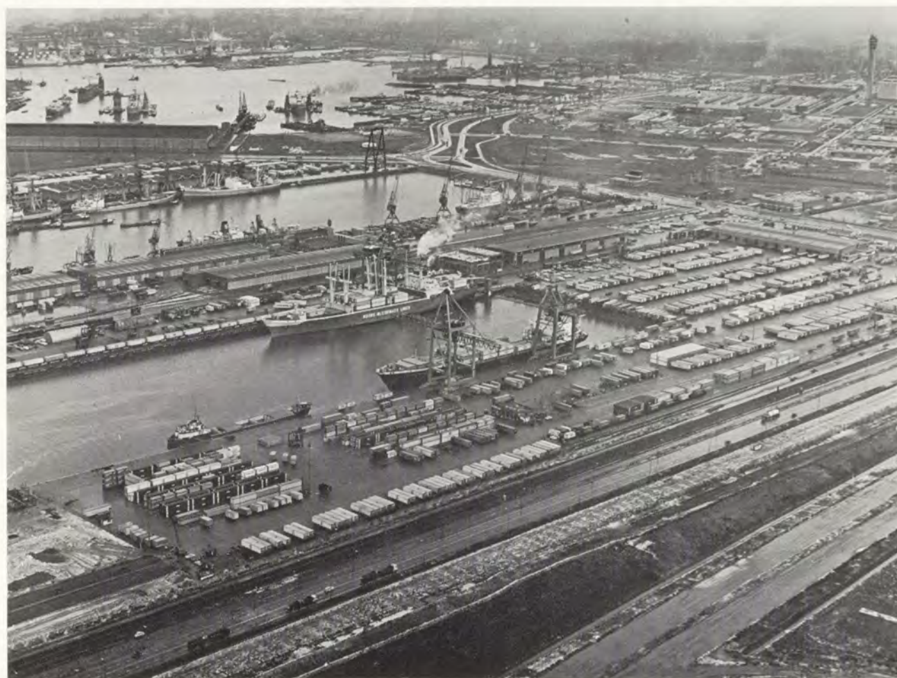
Figure 14 - Infrastructure and facilities of the port must be geared to continual adaptation.
