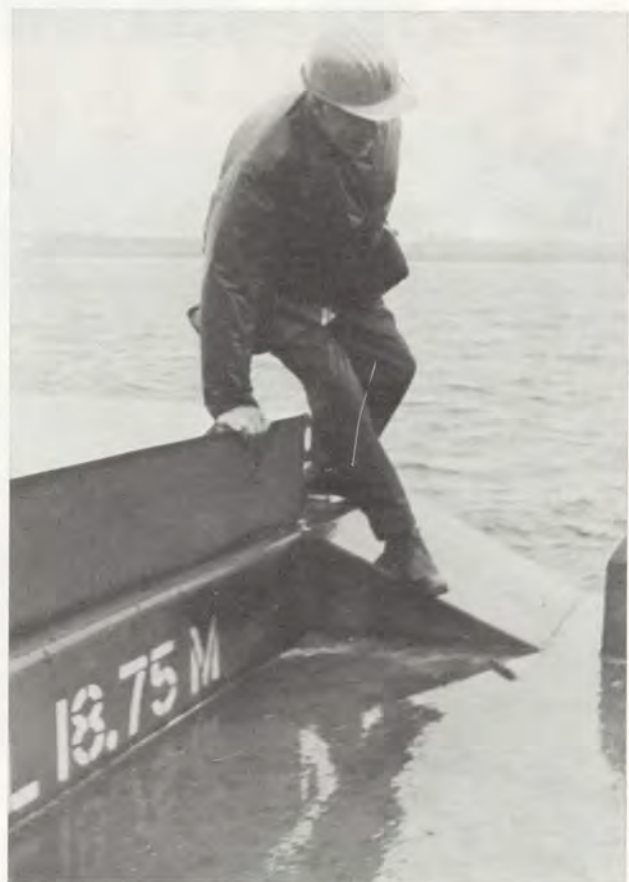
Figure 24 - The barge must be made anti-slip.
