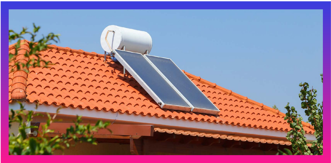
A rooftop thermal solar system (Photo © iStockphoto.com | AlSimonov)
